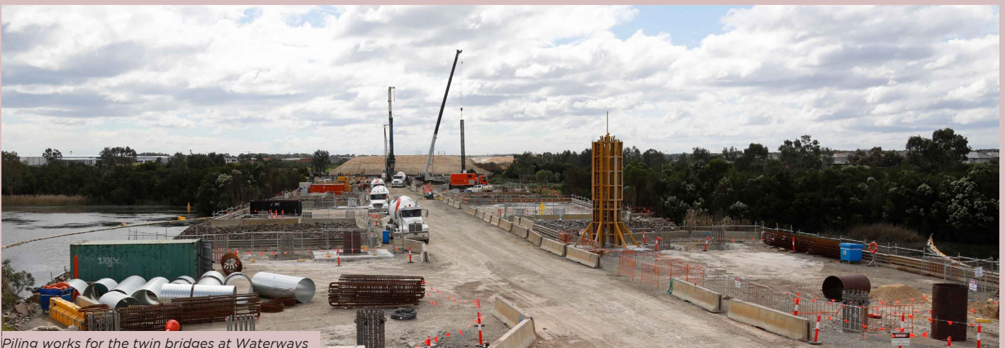
Piling works for the twin bridges at Waterways
